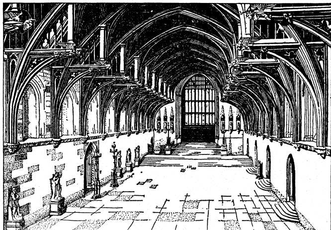
HAMMERBEAM ROOF IN WESTMINSTER HALL. A FINE EXAMPLE OF THE ARCHED TYPE SHOWING ITS GREAT STYLE AND DIGNITY
